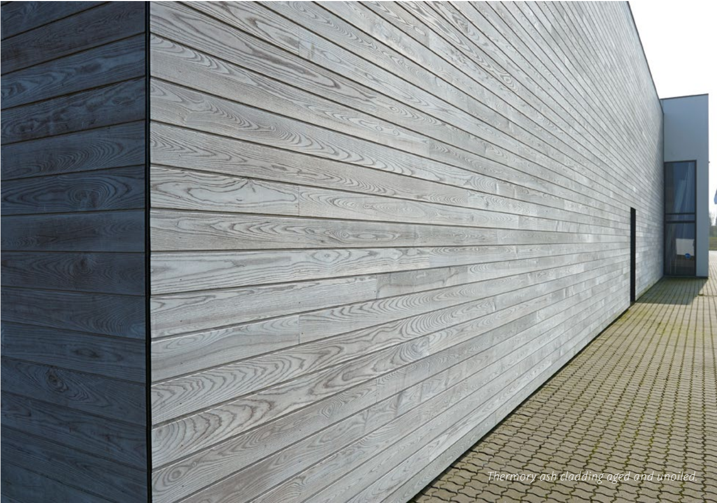
Thermory ash cladding after installation.
